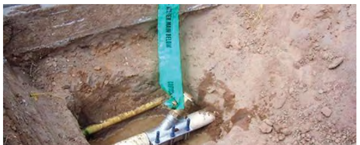
Coliban Water Linestop - Campbell's Creek
