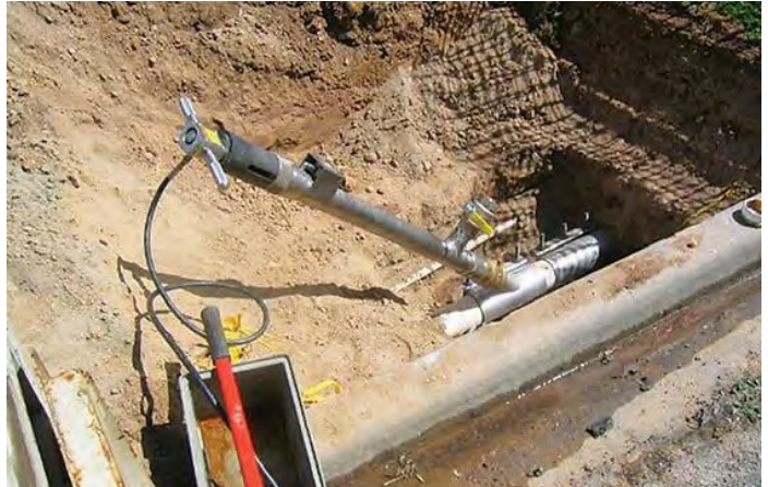
Coliban Water Linestop - Campbell's Creek
