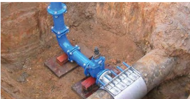
TUP Hydrant Installation at Casterton
